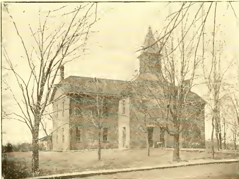
THIRD WARD PUBLIC SCHOOL BUILDING.
